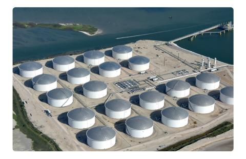
A structurally supported aluminium dome roof is clear span and does not require a supporting column and a fully triangulated aluminium space truss with the structs joined at points on the surface of the sphere. Mario Strache, CEO at Elsont says: 'Aluminium closure panels are firmly attached to the frame members providing watertight sealing using gaskets. The roof is attached to and supported by the tank or concrete wall at mounting points equally spaced around the perimeter of the substructure.'
