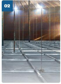
to consider is how the roof configuration influences whether personnel are required to enter the tank in-service to adjust the roof height. With our floating roofs, innovations such as suspension systems allow operators to adjust the IFR position from operating height to maintenance height without putting personnel into a live tank,' says Eickhoff.
