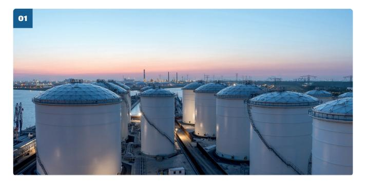
THE ENGINEERING behind each component of a storage tank is meticulously planned to ensure maximum usability for the terminal operator and the workers of a terminal. Tank covers, whether a dome, a roof, or a deck – are no exception. And the style of tank cover will depend on the product being stored.
